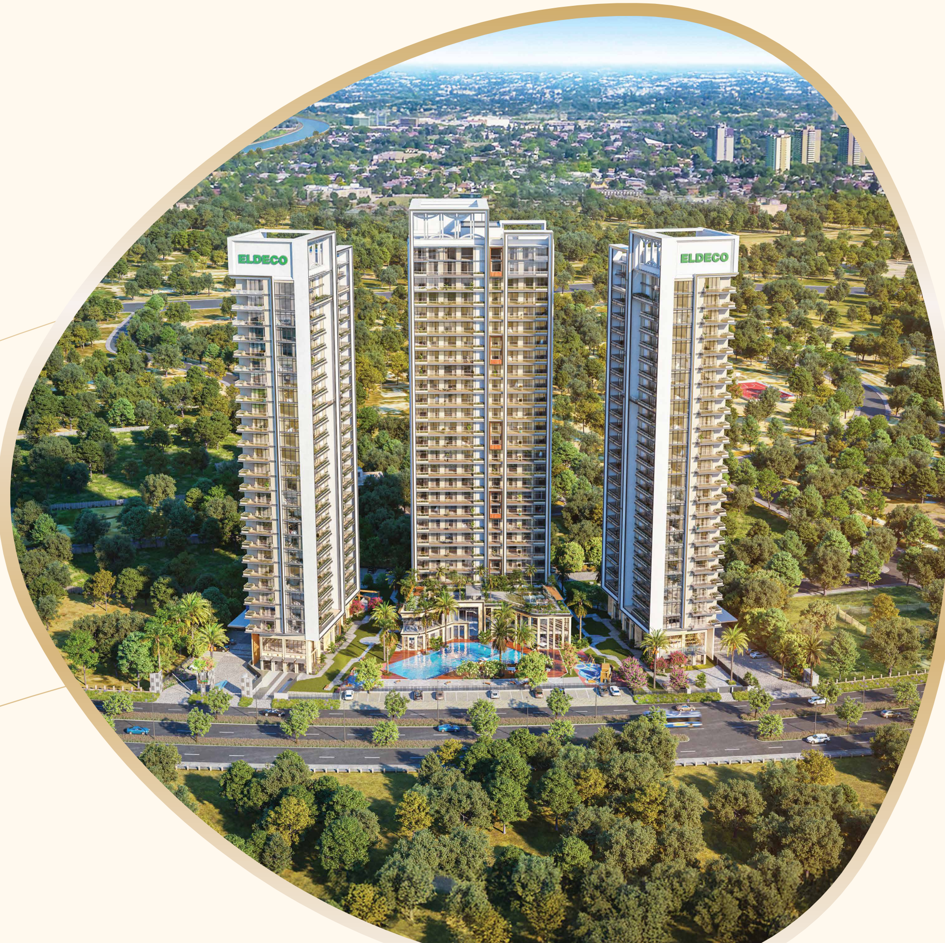
Eldeco Trinity, Gomti Nagar Extension, Lucknow
